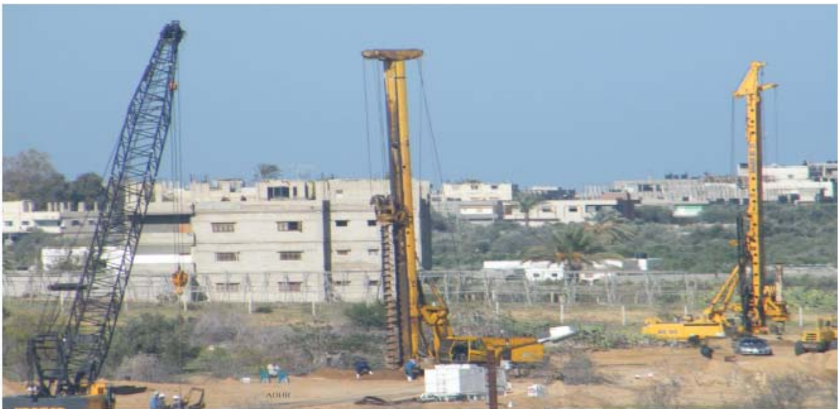
The Egyptian government began instilling the wall of steel at a depth of 20 - 30 metres
