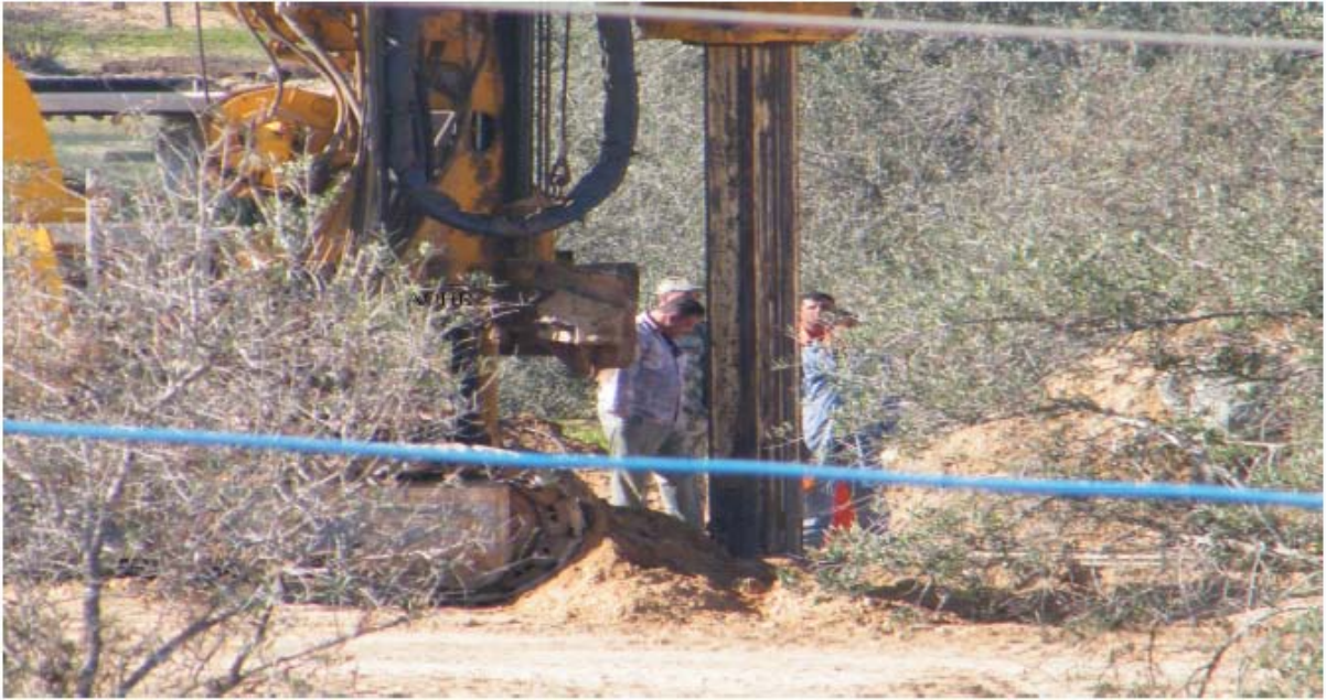
Steel plates for the construction of the wall of shame
